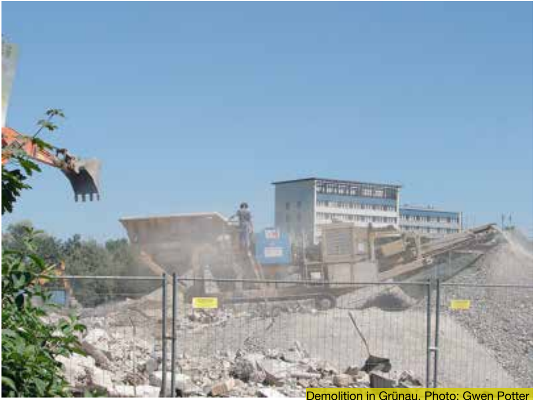
Demolition in Grünau. Photo: Gwen Potter
